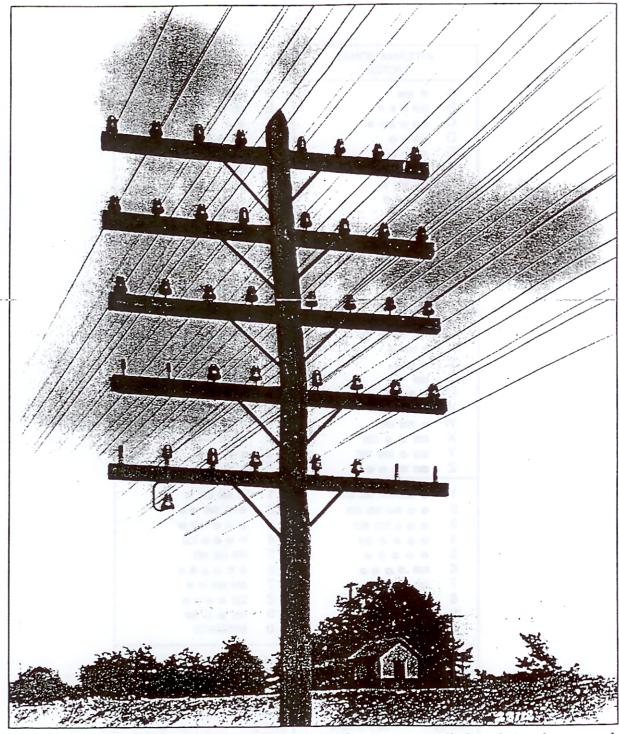
A fine example of a mainline telegraph pole with crossarms filled with insulators and wires. Note the 'roofed' top of the pole to shed rain and snow. The many styles of insulators in common use is prominent. On the pole, wires would be for the dispatcher's circuit, commercial operations (news papers, commercial telegraph, stock tickers etc.) and railway signalling circuits. (CNR Public Affairs, #23112)
